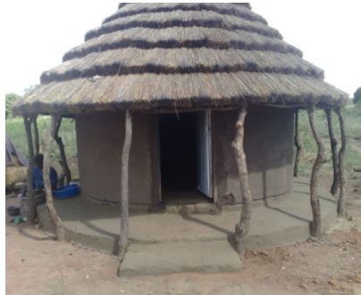
One of the completed huts in Katakwi
