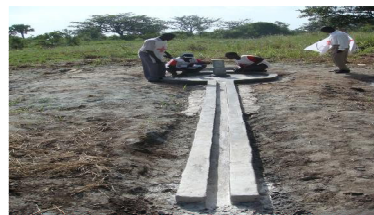
One of the boreholes under construction in Katakwi
