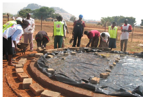
Volunteers help construct a model floods resistant hut in Soroti.
