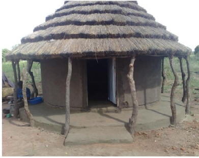
One of the completed huts in Katakwi
