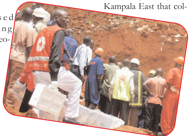
URCS Kampala Central volunteers at the excavation site on Lumumba Avenue, Kampala.
